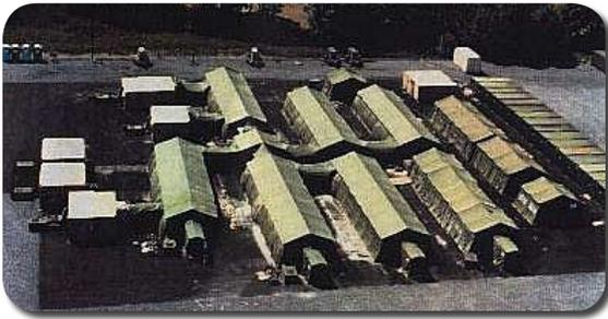
The Army's CP DEPMEDS program is a Joint effort to insert environmentally controlled collective protection into currently fielded hospital shelters. The requirement is to be able to sustain medical operations for 72 hours in a chemical contaminated environment. Environmentally controlled collective protection is
