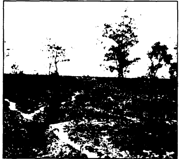
(U) Udorn site before construction started in 1965
