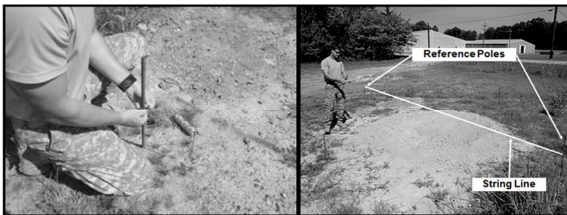
Figure G-9. Step 2. Establish reference data points
