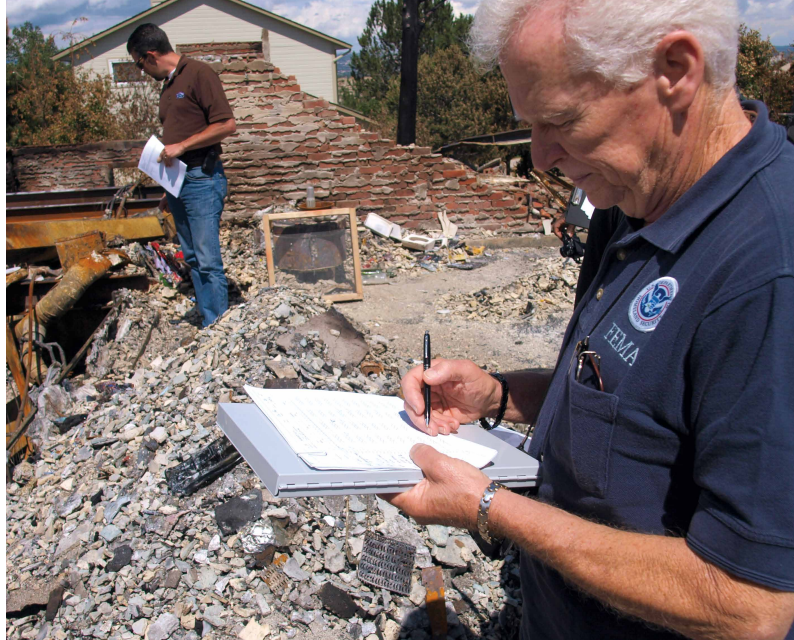
Assessing damage from the Waldo Canyon fire in Colorado. Source: FEMA Photo Library
