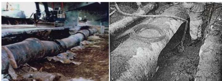
Figure A-4. These photos show some of the effects of earthquakes on buried pipelines. (left) Ductile iron pipes with seismic joints can survive large ground deformations. (right) Cast iron pipes can undergo brittle failure.
