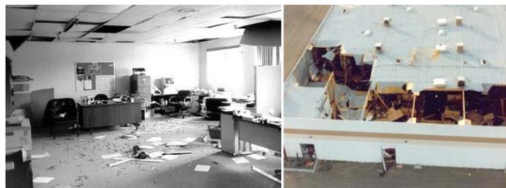
Figure A-11. Images of blast damage at Henderson, NV, courtesy of the City of Henderson, NV, similar to that expected at the outer edge of the LDZ.
