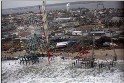
Source: GAO analysis of National Security Council documents, White House (photo). | GAO-15-20. Damage of New Jersey's barrier beaches.
