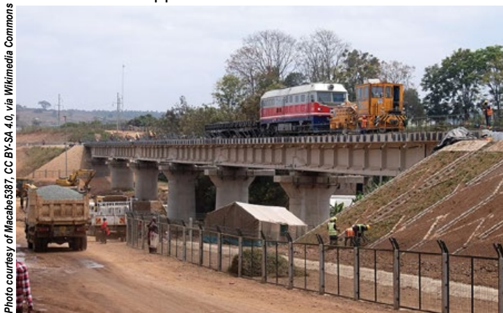
A DF4D diesel electric locomotive owned by the China Road and Bridge Corporation is parked on a bridge construction site of the Nairobi-Malaba Standard Gauge Railway Project in Kenya.
