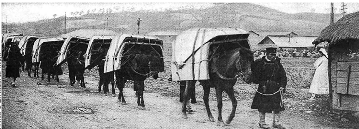
Japanese Pontoon train moving to Yalu River from Ping-Yang. Pontoons were built in Hiroshima before the outbreak of the Russo-Japanese War in 1904 in preparation for crossing the Yalu River. The sections were later transported via horse teams.
