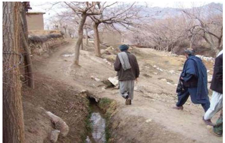
An example of where a small irrigation efficiency project could benefit rural villagers. Installing a concrete structure would replace the present wood/stone structures installed for crossing of the channel. It is very difficult to maintain the interiors of the current structures.
